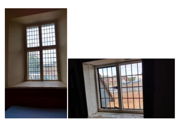
The hinged windows in the hall and upper room should be kept maintained. Small draughts can be blocked by use of black plasticine (recommended by Historic England) – it can fill small to medium gaps and is easily removed.
