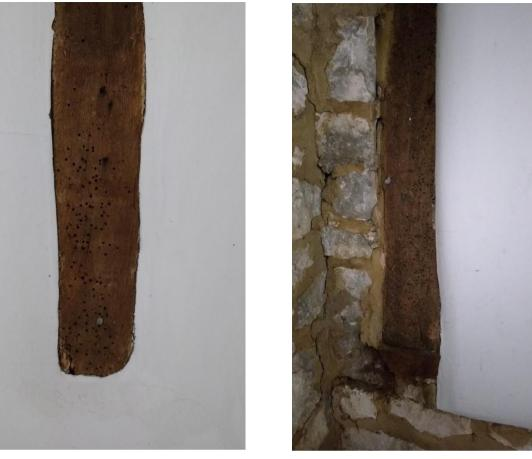
Evidence of past attack from wood boring beetles is seen in the end first floor room. No evidence of recent activity (i.e. sawdust) was noted. A watch should be kept for beetle activity, especially in rarely viewed spaces such as inside cupboards and the underside of furniture. Small infestations can be dealt with using a handheld sprayer, whereas large problems such as under floors or in the roof structure require professional treatment.
